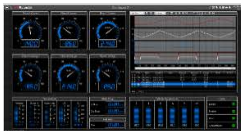
SRB Control PLC SCADA
